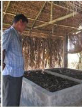
Getting encouraged, farmers started to construct cemented tank
